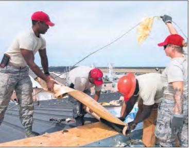
Airmen from the 823rd Red Horse Squadron, Hurlburt Field, Fla., lay insulation on a hangar roof Oct. 22 at Tyndall Air Force Base, Fla.
